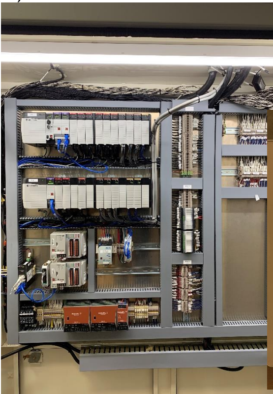
Photo 1- CVWPCC PLC Rack
