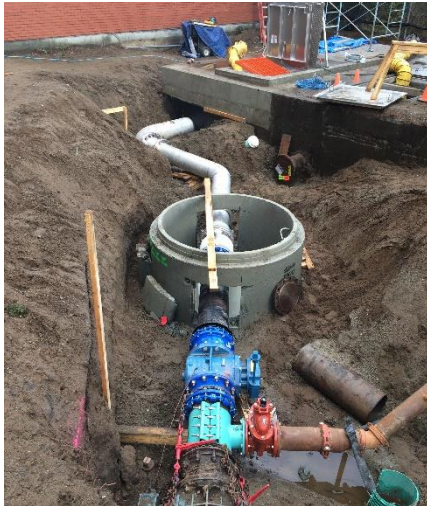
Photo 1- New piping, flow meter and valves
