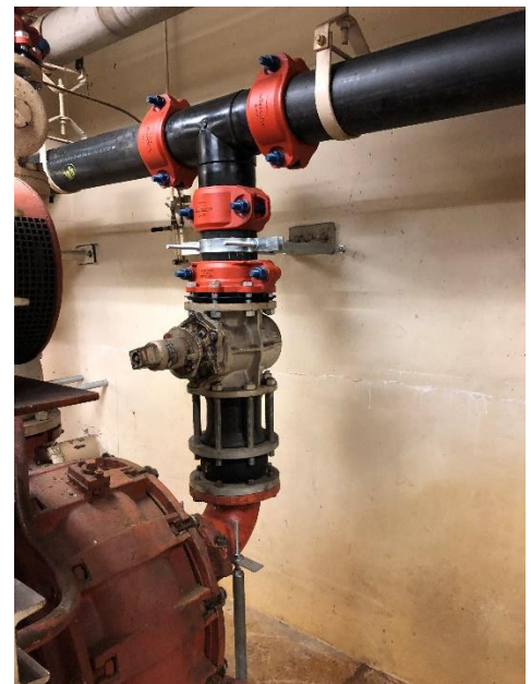
Photo 2- Basement piping, primary sludge lines replaced.
